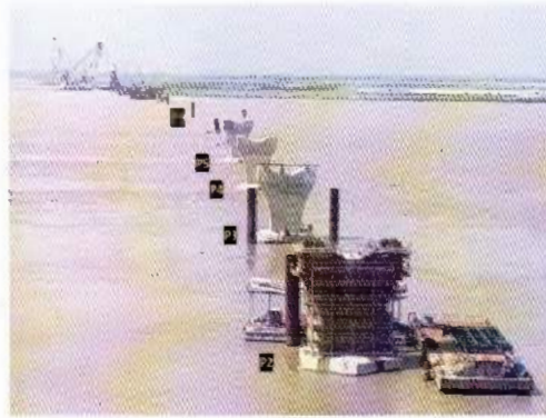
Overall activities of Pier and Pile Cap at Mawa site
