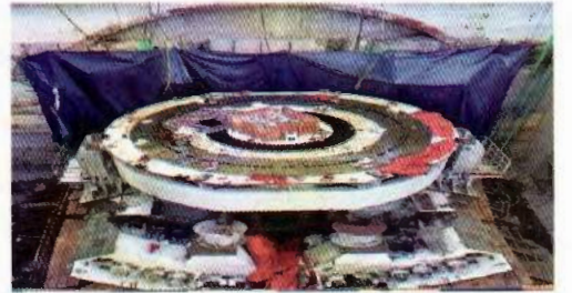
TBM main drive being assembled in the LB
