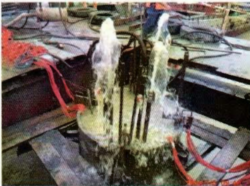
Anchor Pile Driving for TD4B
