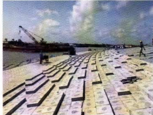
CC Block Production River Training Works Activities
