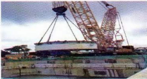
TBM main drive being hoisted into the LB
