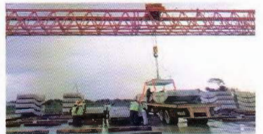
TBM segments arrived at the site
