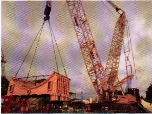
TBM steel sleeve pedestal being hoisted into the LB
