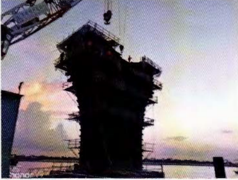
Pile Cap, Pier Shaft & Pier Cap
