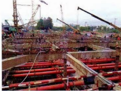
C&C section construction site
