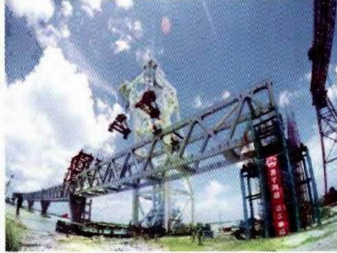
5 th span erection
