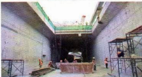
West bank C&C section left route wall repair
